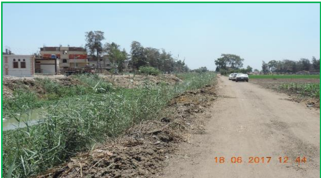
Figure 4-3: shows Mit AL Amel drain within Qarmut Al Bahw village in Aga district.
