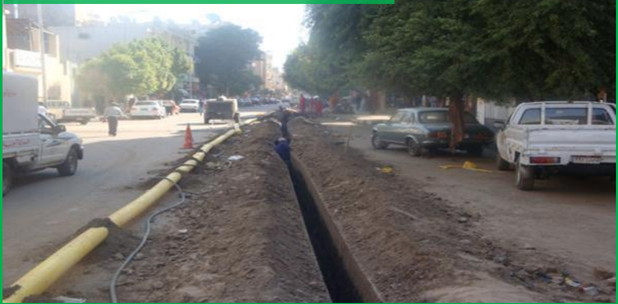
Figure 2-24: Pictures showing sample of typical trench for PE pipes by Egypt Gas
