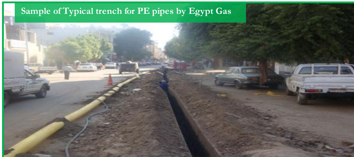
Figure 2-4: Picture showing sample of typical trench for PE pipes by Egypt Gas
