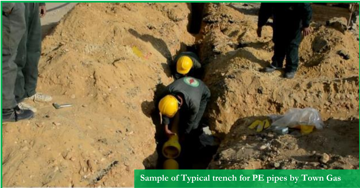
Figure 2-42: Pictures showing sample of Typical trench for PE pipes by Town Gas
