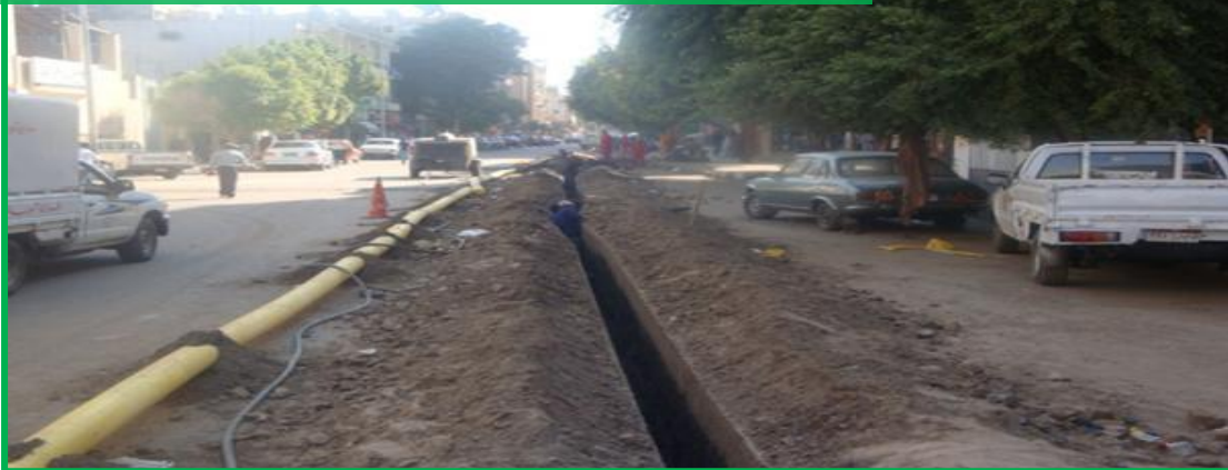
Figure 2-4: Picture showing sample of typical trench for PE pipes by Egypt Gas
