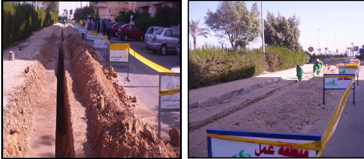
Figure 2-22 Typical trench for PE pipes
