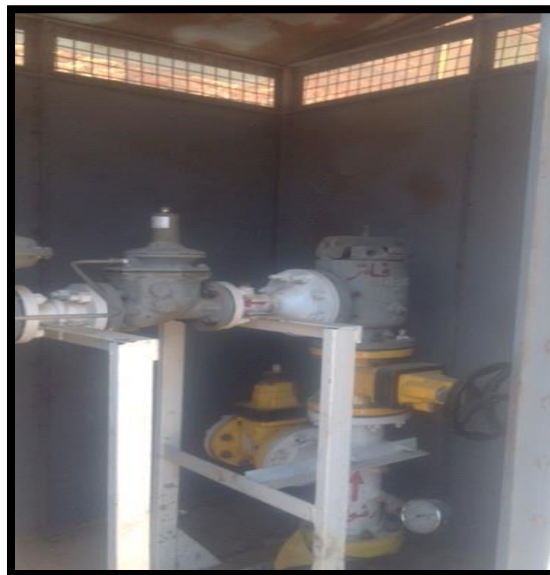
Figure2-5 Example of Cairo Gas pressure regulators
