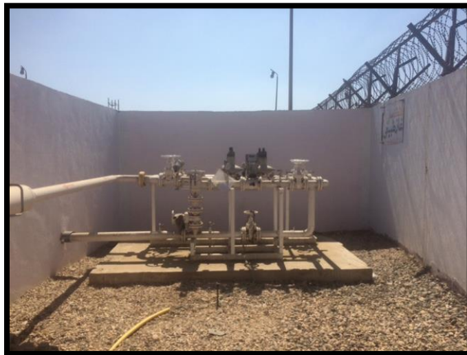
Figure2-7 View of the existing pressure reduction station affiliate to GASCO
