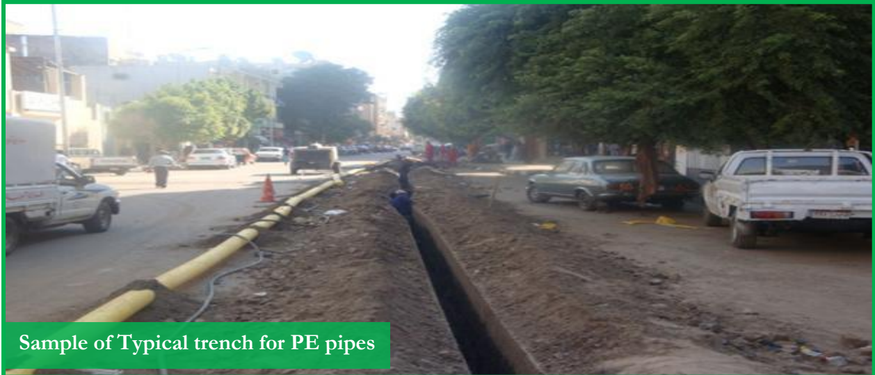
Figure 2-12: Picture showing sample of typical trench for PE pipes
