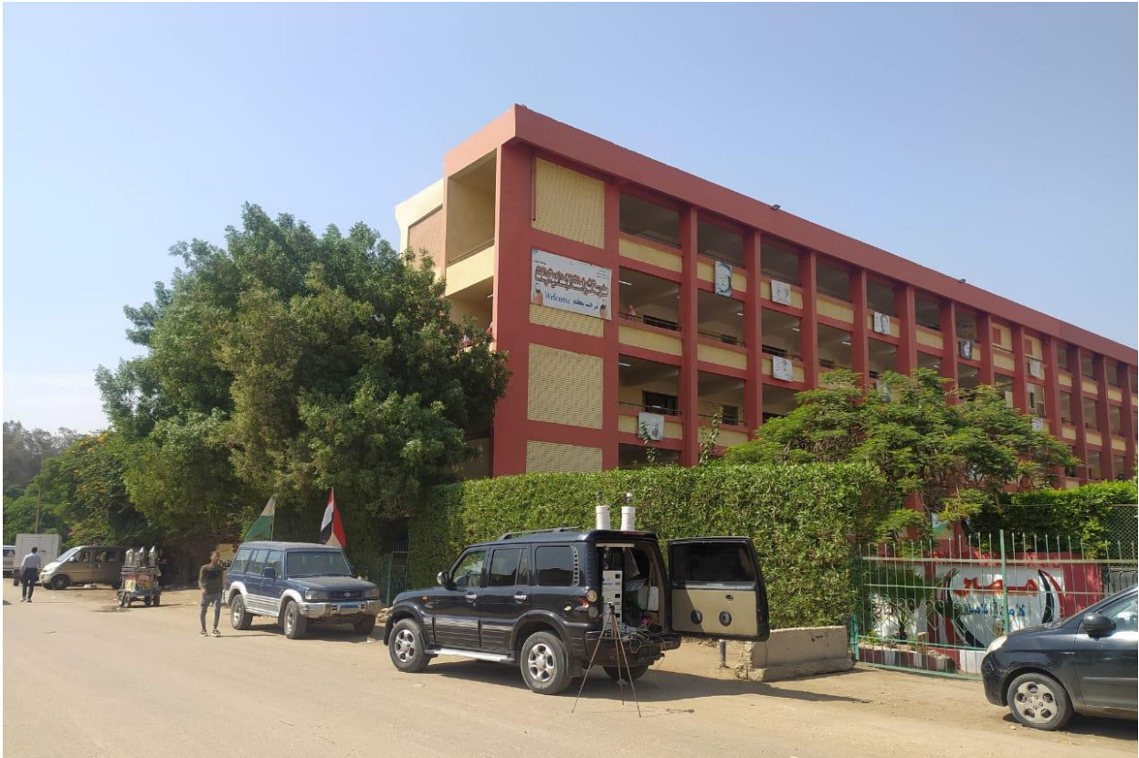
Figure 3-1 ambient air quality monitoring system and noise measurements
