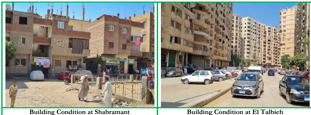
Figure 4-7: Pictures showing Building Condition at Shabramant and El Talbieh.
